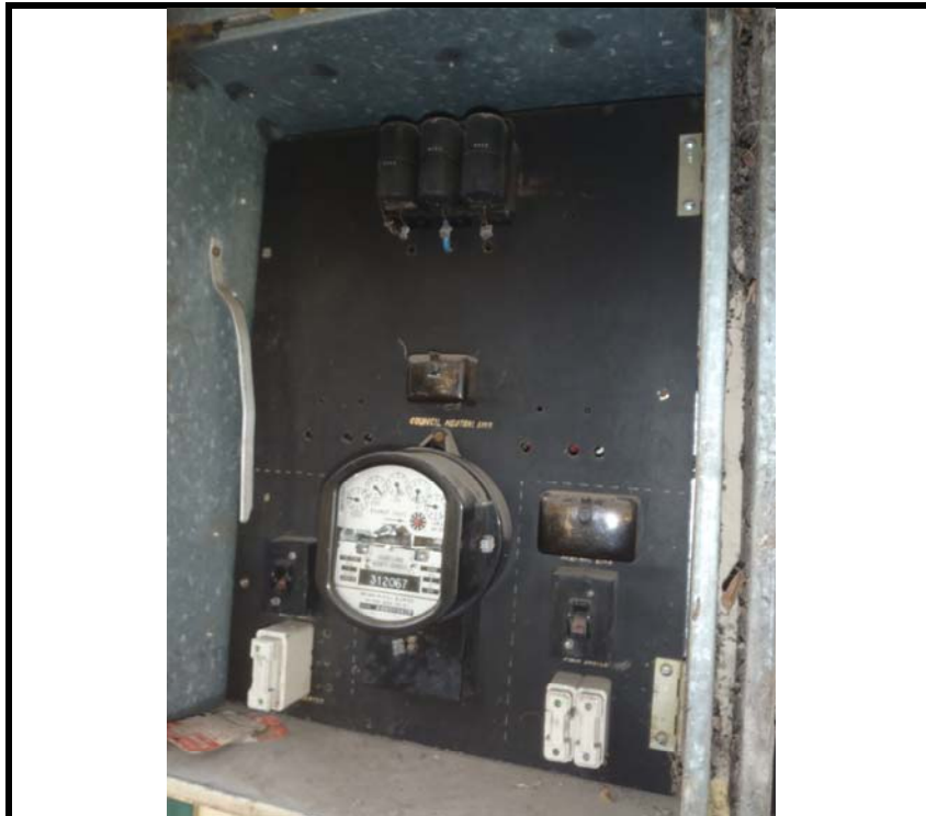
Photo 14: One of the two ACM zelemite backing boards in power boxes attached to Unit 1A at 1 McLeod Road.
