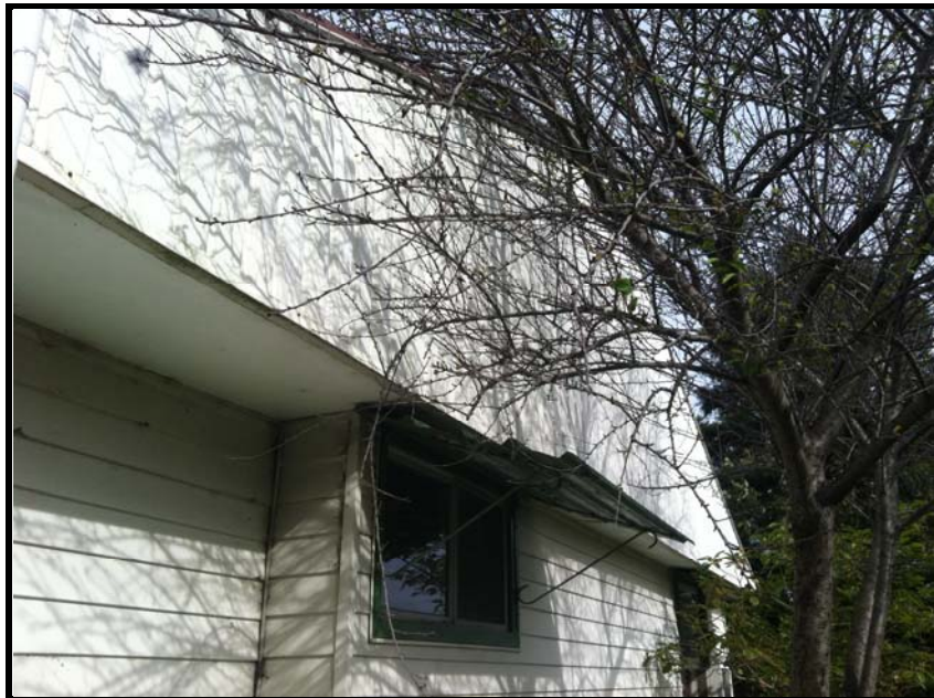
Photo 22: Example of the vinyl veneer used on the gable end and exterior walls to the main house at 5 McLeod Avenue. The veneer appears to cover ACM sheeting. The photo also shows ACM sheeting used for the eaves.
