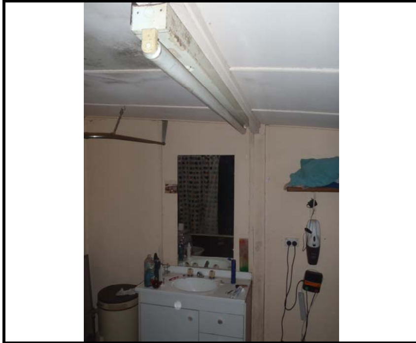
Photo 15: ACM sheeting to the walls and ceiling, and potentially PCB-containing fluorescent light in the bathroom area of Unit 1A at 1 McLeod Road.
