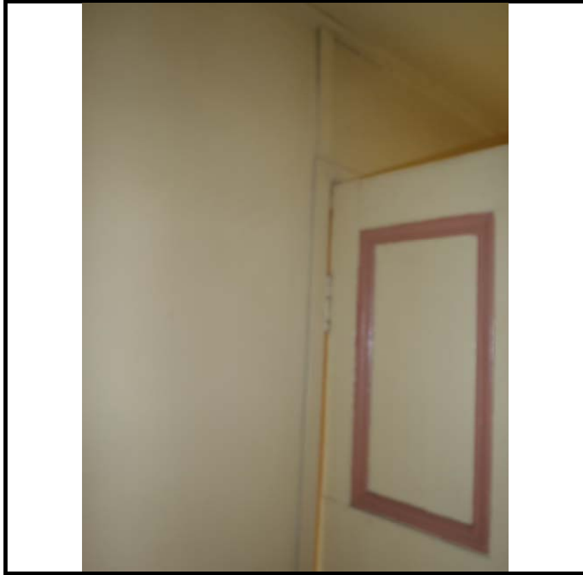
Photo 9: Some of the ACM sheeting used to the side and above the back door at 1 McLeod Road.
