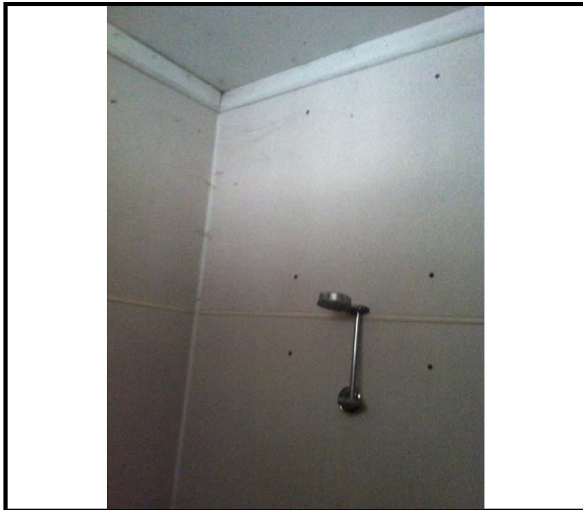
Photo 30: ACM sheeting (patterned) to walls and to the ceiling in the shower area of the brick section of 5 McLeod Road. ACM sheeting also used in the ceiling of the adjoining toilet room.
