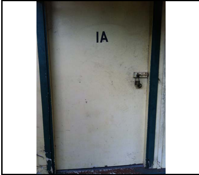
Photo 17: ACM sheeting attached to timber frame used for front door to Unit 1A at 1 McLeod Road.
