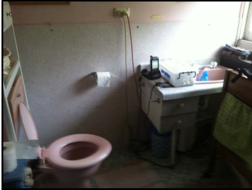
Photo 23: ACM sheeting (including lower section with pattern print) in walls to bathroom section of front room of 5 McLeod Road.
