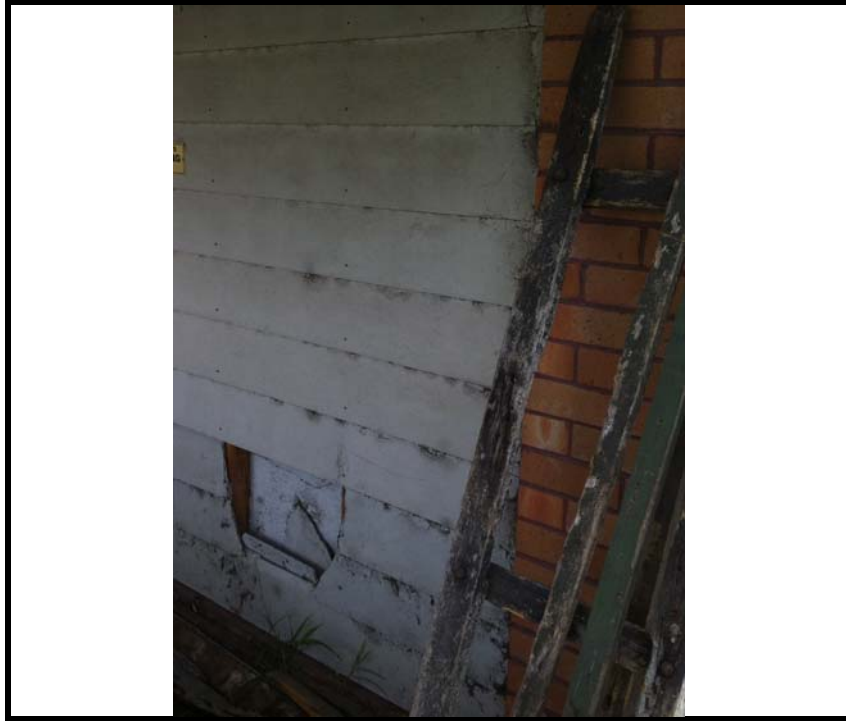
Photo 31: panels used as infill to a former garage entry to the brick section of 5 McLeod Road. Laboratory analysis concluded these are not ACM.
