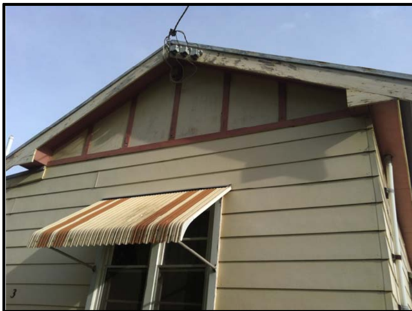
Photo 19: ACM sheeting used in gable end , eaves and exterior wall panelling to 3 McLeod Avenue.
