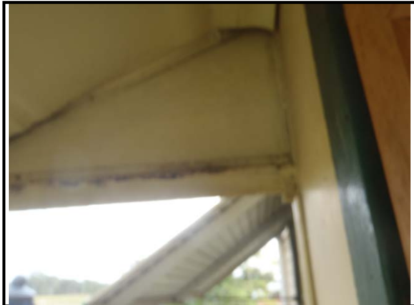
Photo 10: One of the side panels constructed of ACM sheeting to the side of the back door awning at 1 McLeod Road.
