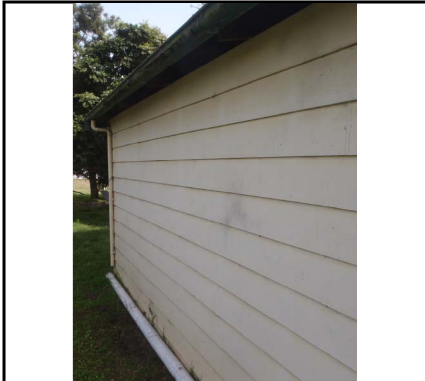
Photo 12: Panels to exterior walls of the garage at 1 McLeod Road. Laboratory analysis concluded these are not ACM.
