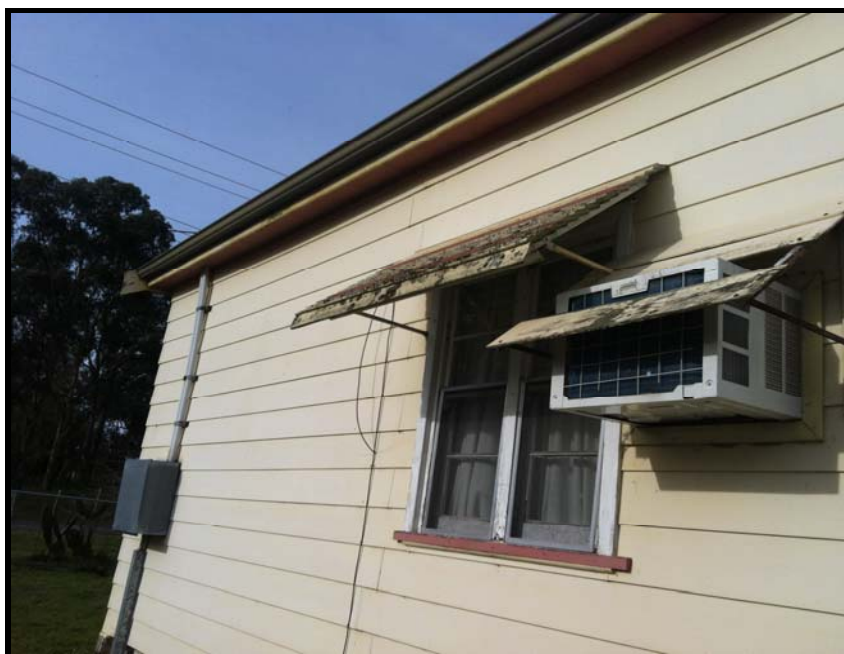
Photo 20: ACM sheeting used in exterior wall panelling to 3 McLeod Avenue.
