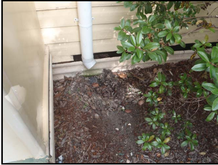
Photo 3: Section of the ACM corrugated sheeting used between the garden bed and under the house and Unit 1A at 1 McLeod Road.
