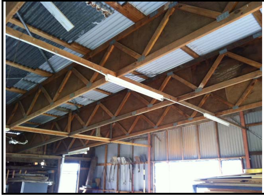
Photo 21: Potentially PCB-containing fluorescent lights used in the large shed at 3 McLeod Road.
