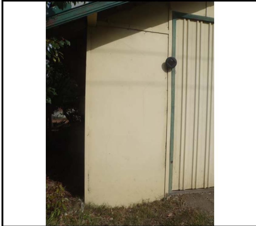
Photo 13: ACM sheeting exterior wall panels to Unit 1A at 1 McLeod Road.
