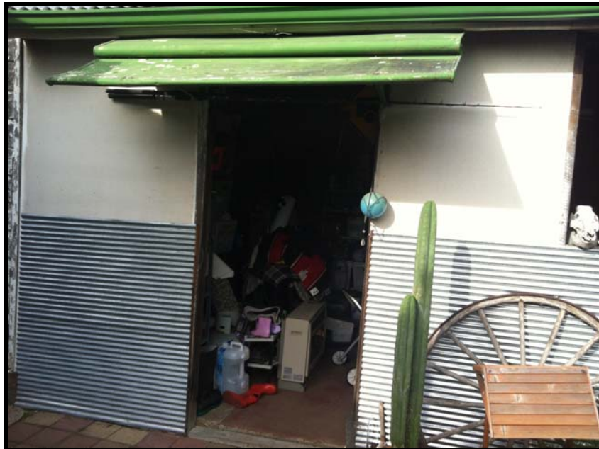
Photo 28: ACM sheeting (including behind corrugated iron) used to the side of the outdoor area at the rear of garage at 5 McLeod Road.
