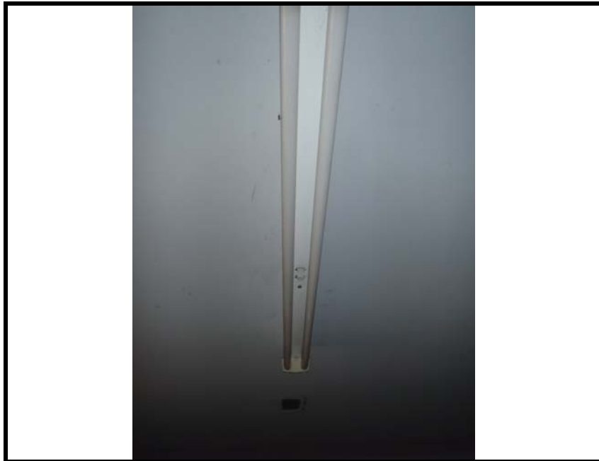
Photo 18: One of the potentially PCB-containing fluorescent light in the general area of Unit 1A at 1 McLeod Road.
