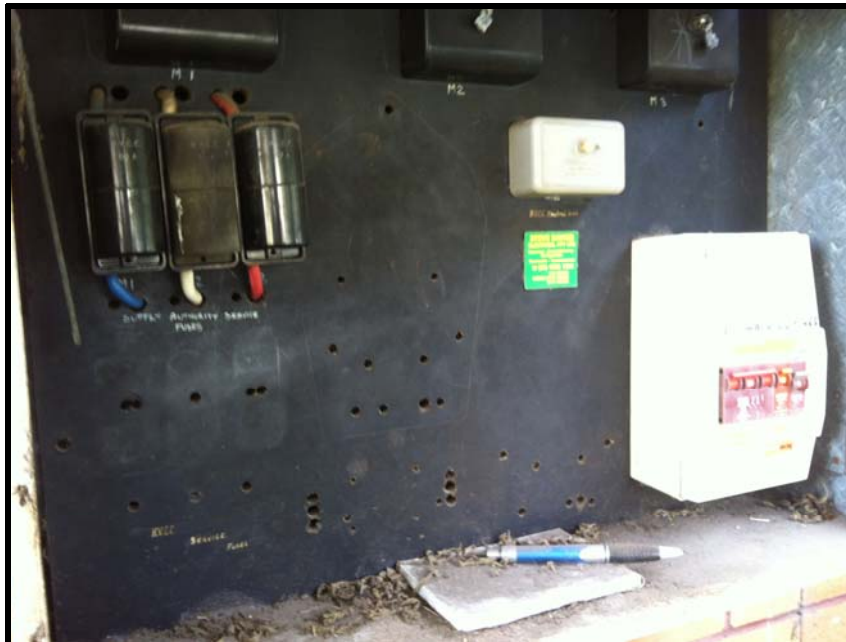
Photo 32: ACM zelemite back board to power box attached to the brick section of 5 McLeod Road.
